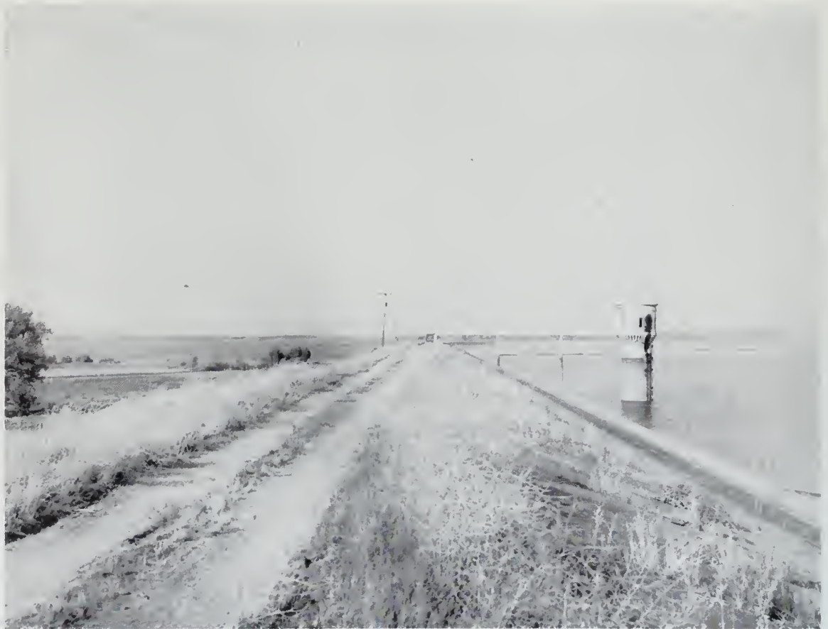
Woodward Dam on Simmons Creek
